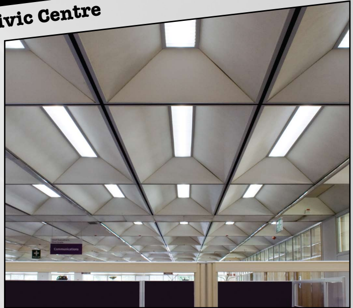
New LED Lighting
